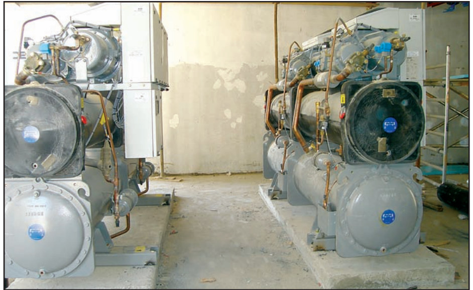
PCS's absorption chiller system uses hot water to provide cooling to the building. Water pipes run through the solar panels providing 95% efficiency in terms of hot water production.
